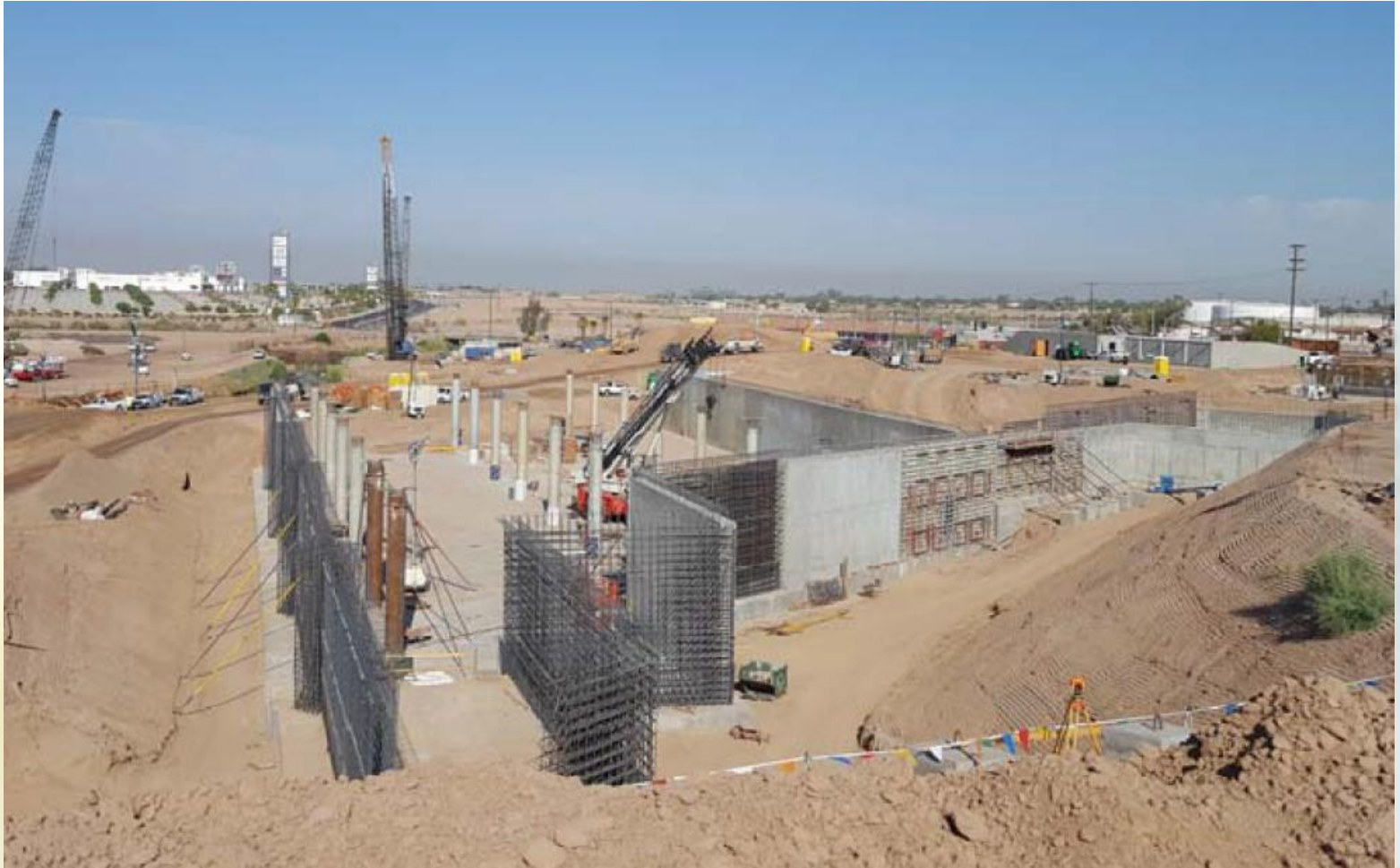
Looking north – Shell Space structure
