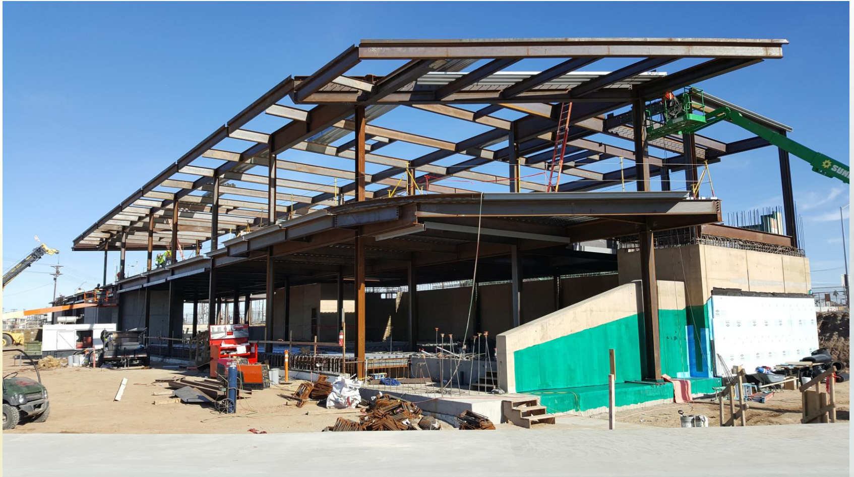
Looking north – new Headhouse
