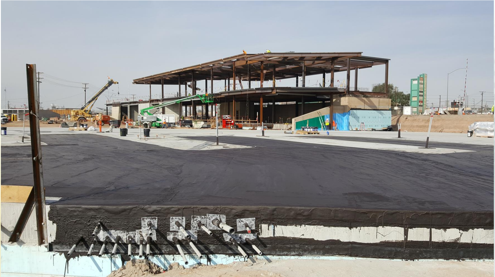
Looking north – northbound POV inspection
