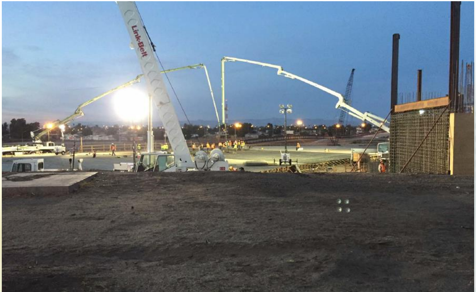
Looking north – concrete pour of Northbound POV lanes
