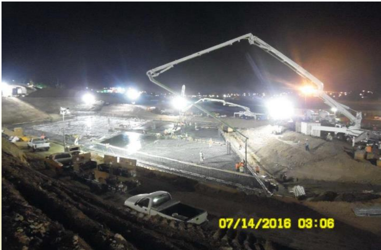
Looking south – concrete pour of Shell Space slab
