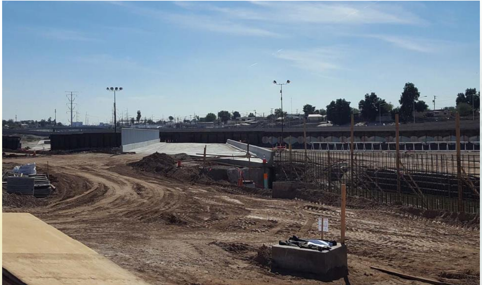
Looking south towards Mexico – Southbound POV across new bridge
