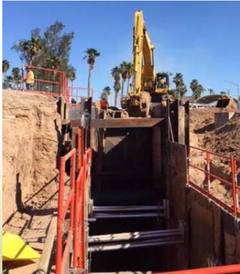
60" Storm Drain Line Installation
